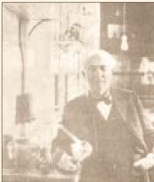
Edison with two of the electric bulbs which in 1880 produced the 'Edison effect' - the outflow of electrons into vacuum from a heated conductor. (Also known as thermionic emission)
